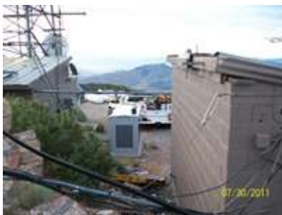
The Repeater Site
