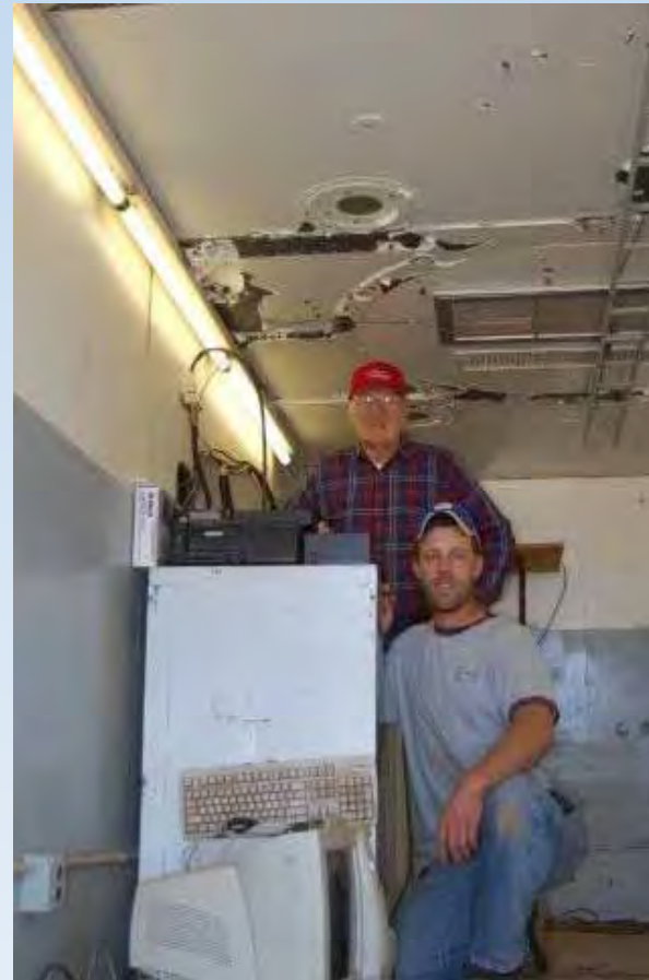
Casey and Bill Wells (W7WFW) Installing 45 Repeater Hardware
