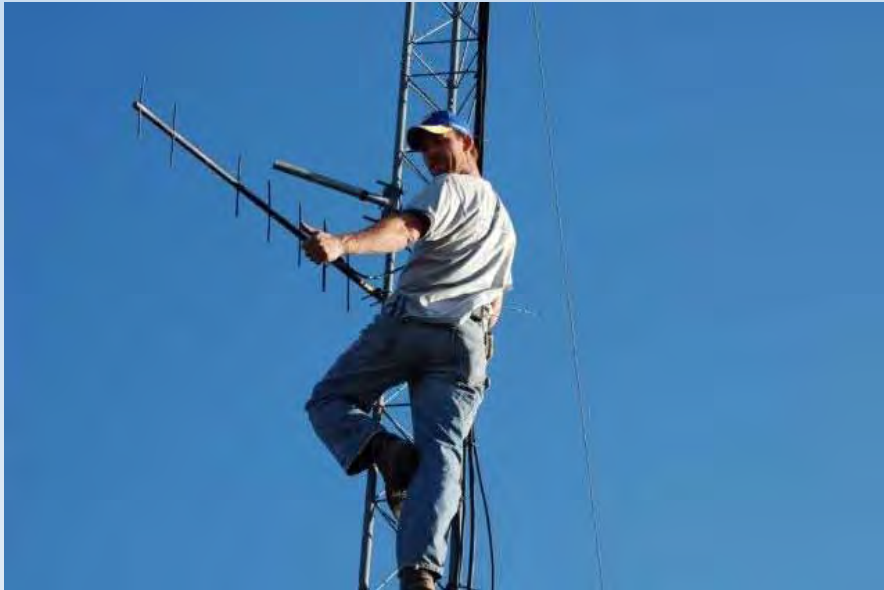
Casey Lofthouse (KD7HUS) Installing 45 Repeater Link Antenna
